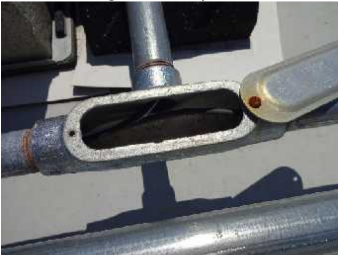
Exhibit 5. Missing Conduit Body Gasket
