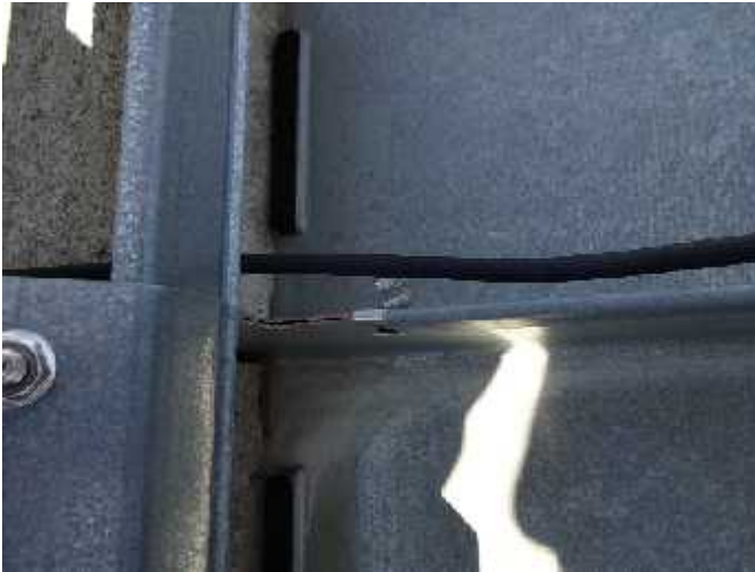
Exhibit 5. Missing Conduit Body Gasket
